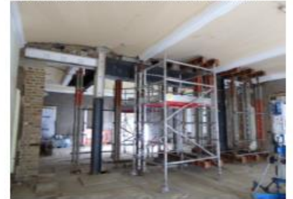
5.14 Removal of needles and props in progress in room 04-024 Wed 16 March
