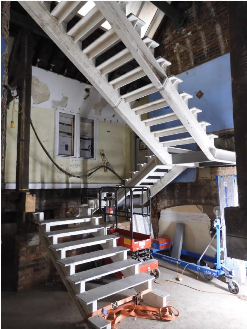
5.8 New stair S20 at level 5 Tuesday 26 July 2022
