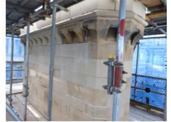
5.87 Chimney CS21 viewed from south-west Tuesday 7 June 2022
