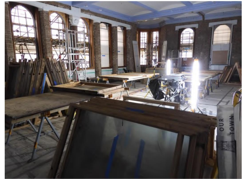
5.39 Sash window repairs and preparation for painting in room 01-019
