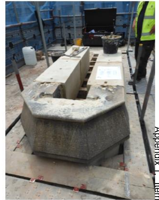
5.90 Top of chimney CS21 viewed from north Tuesday 7 June 2022
