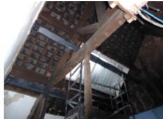
5.11 Steel beams installed on north side of Lloyd Street roof
