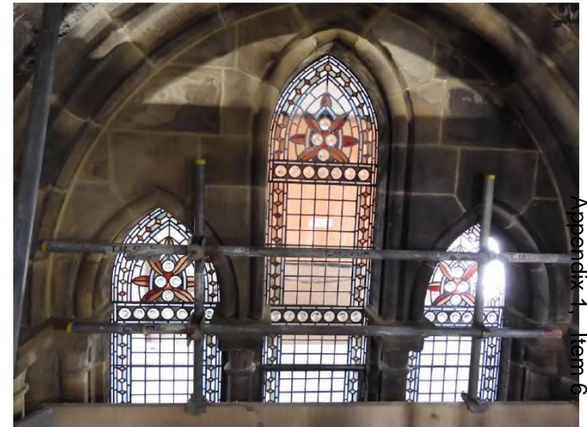
5.46 View of leaded lights re-fitted in level 2 corridor from Princess St courtyard
