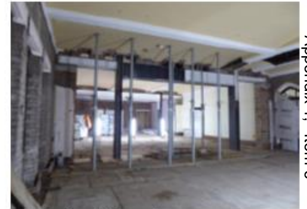
5.16 Overview of room 04-024 from south-east corner
