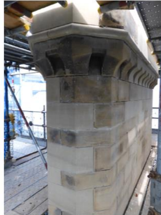
5.88 Chimney CS21 viewed from south-east Tuesday 7 June 2022
